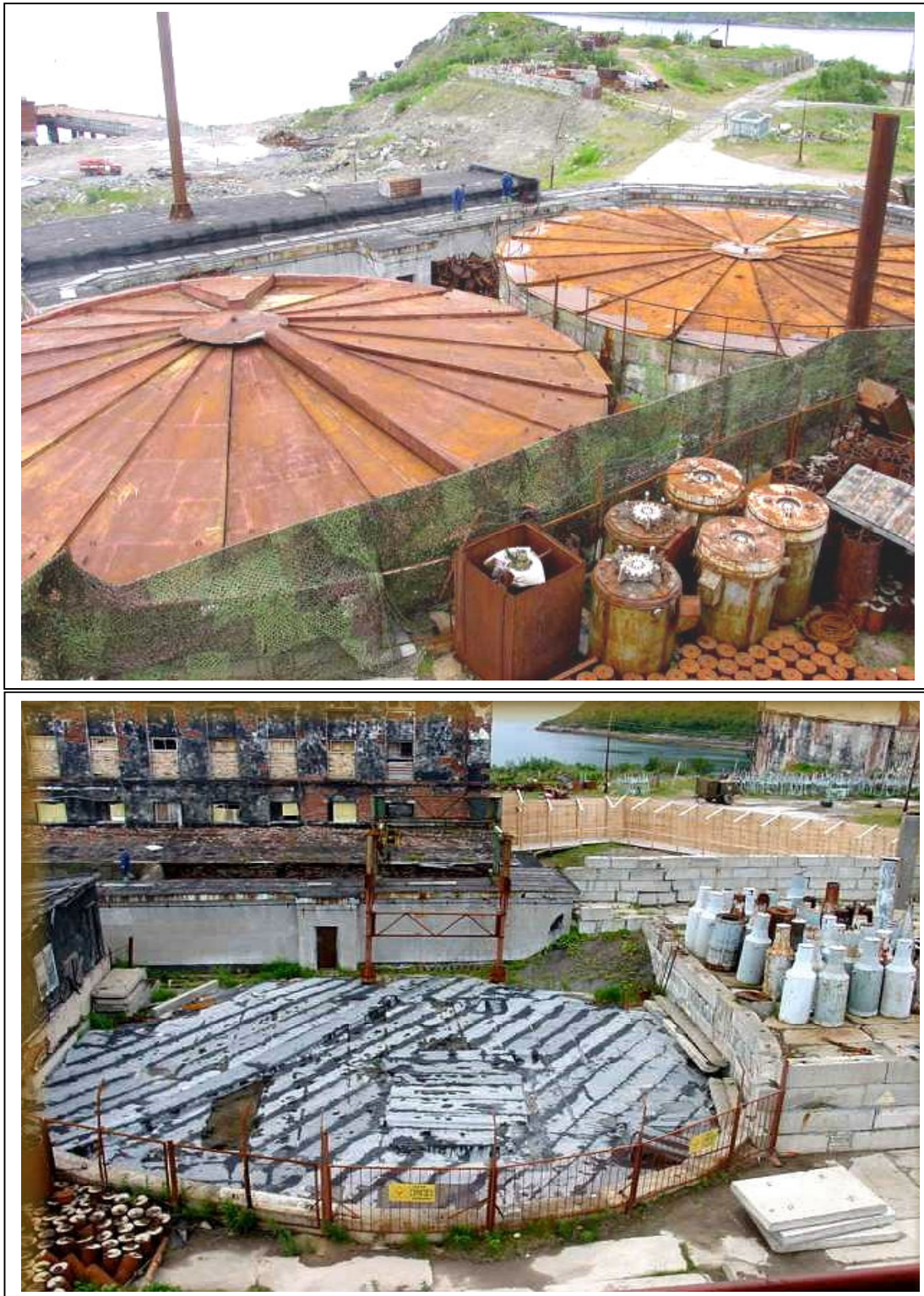
Figure 2.1.1-2. Spent nuclear fuel stores at Andreeva Bay. Facilities 2A and 2B (top) and 3A (bottom)
