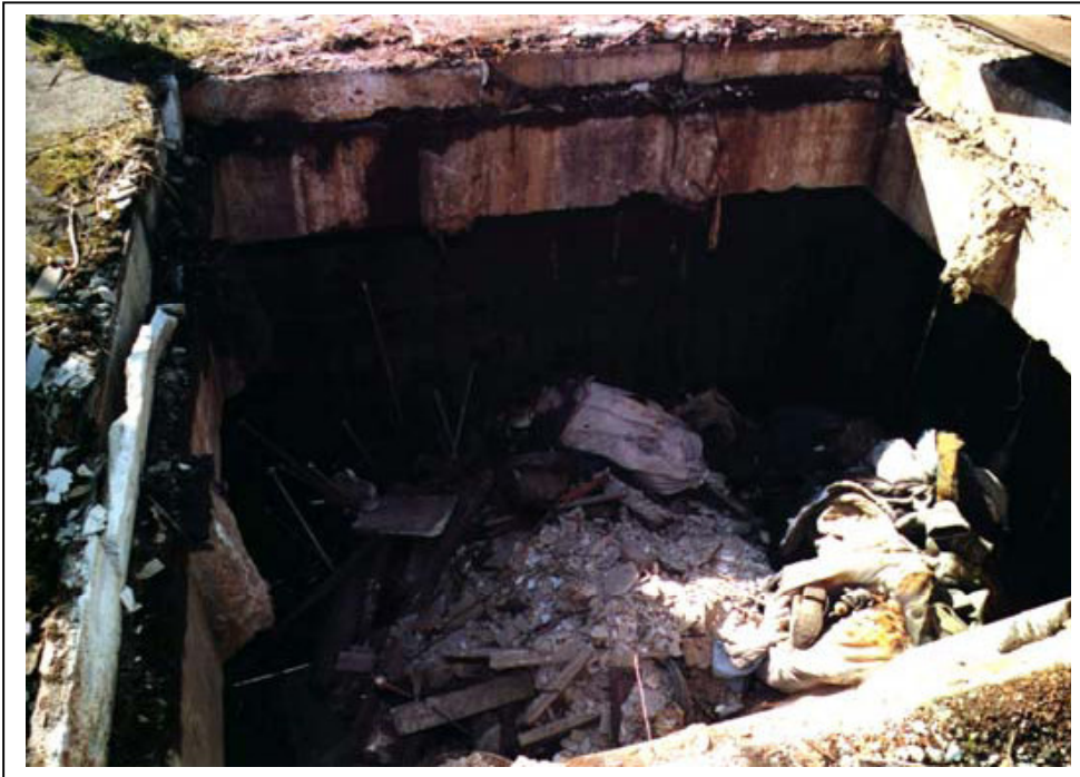
Figure 2.1.4-5: Unpackaged solid radioactive waste within Building 162 at Zvezdochka shipyard
