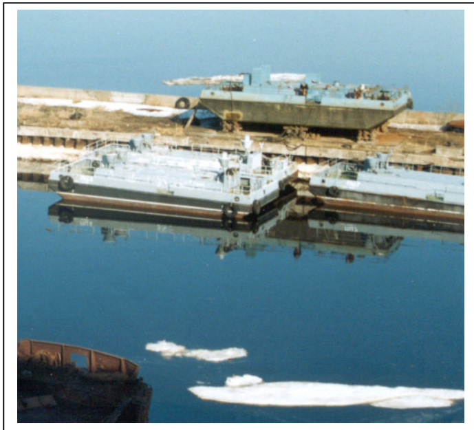
Figure 2.1.5-2. PEK-50 liquid waste storage tanks moored at Sevmash
