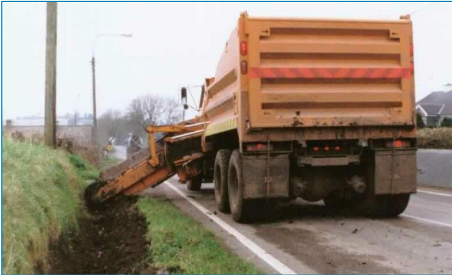
Picture 7 Construction of an open canal on areas where the route
