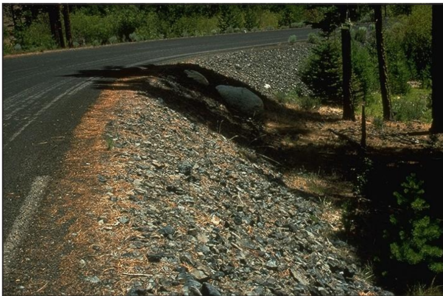
Picture 6 Cladding an embankment with gravel and stone
