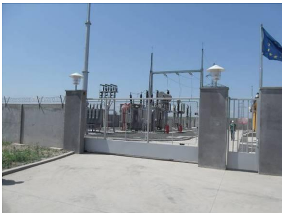
Figure 5: Control building at Wind Farm site.
