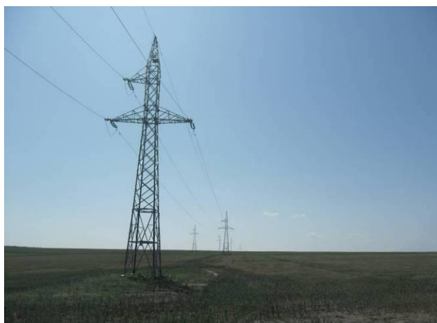
Figure 7 – View of transmission line
