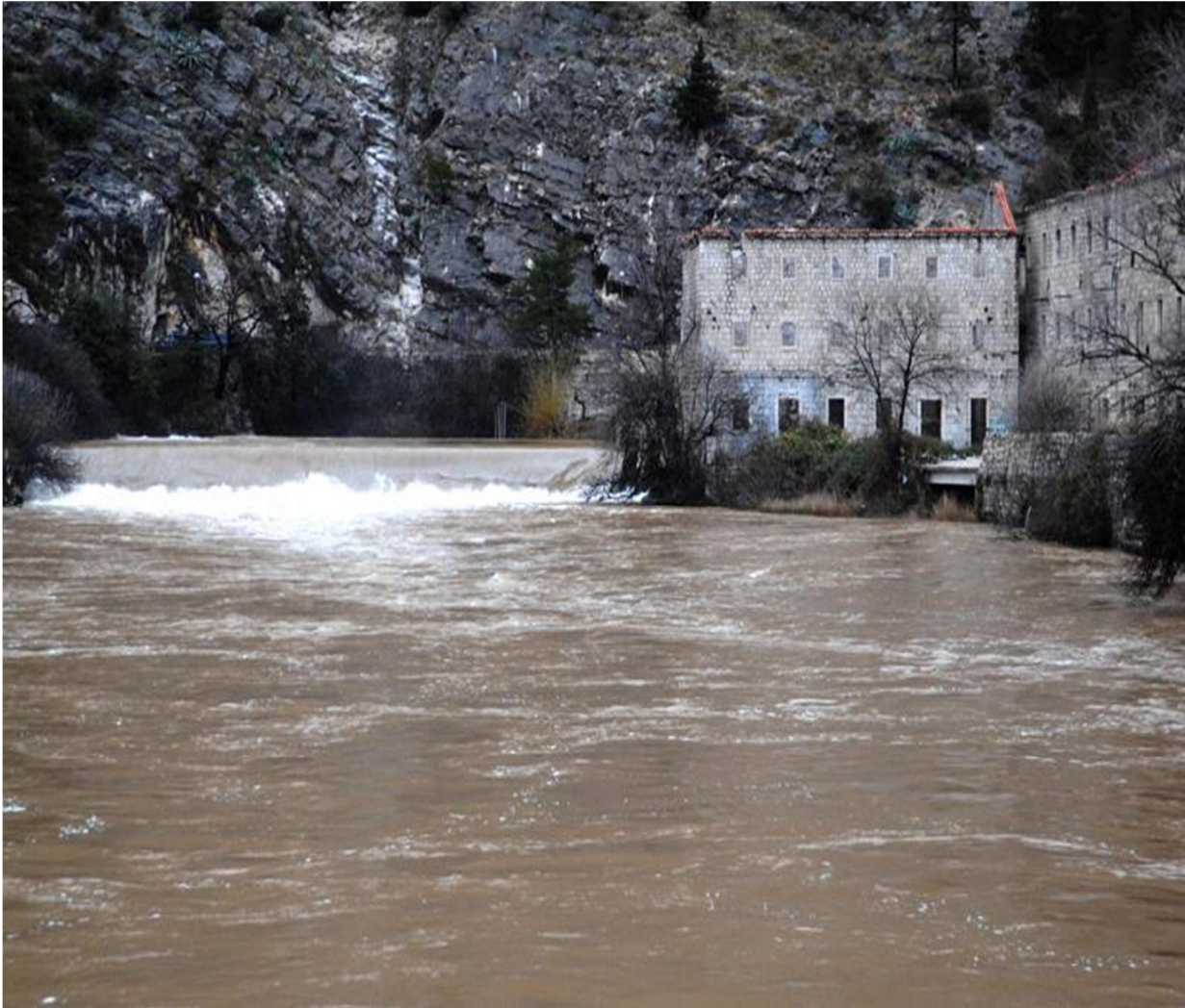
Plate 2: Ombla Spring and Komolac Weir in Flood
