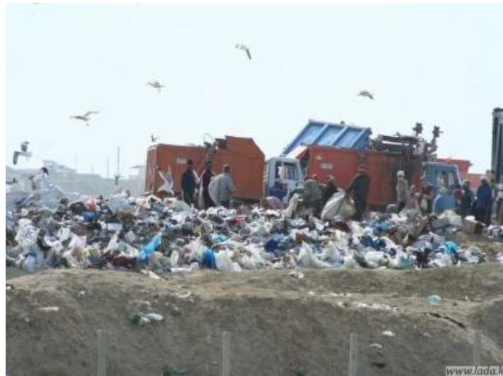
Figure 2. The existing dumpsite (Source: Lada newspaper on internet)
