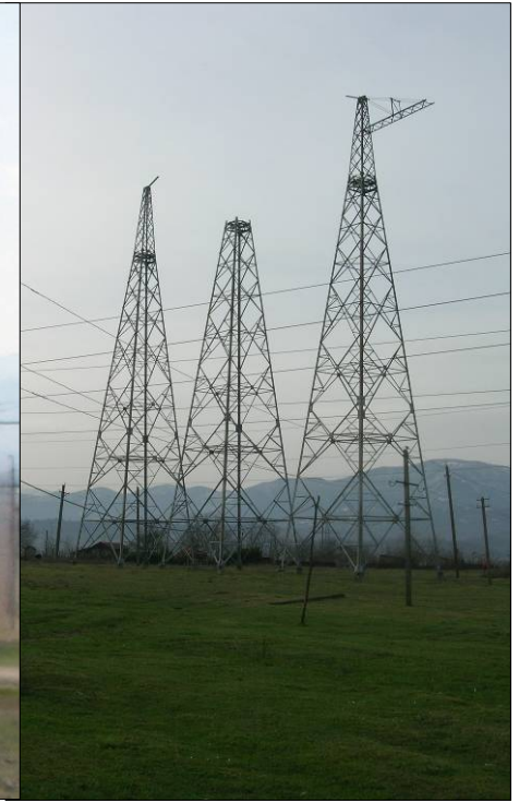
Triple 4-point contact steel lattice towers. Used primarily for direction changes and high conductor stress situations.
