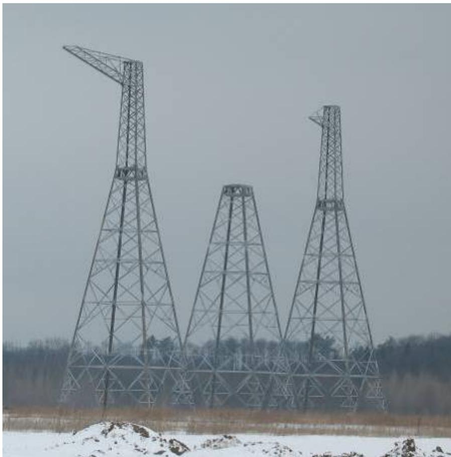
**Figure 6.1** Typical 750 kV angle-tension tower YC750-1
