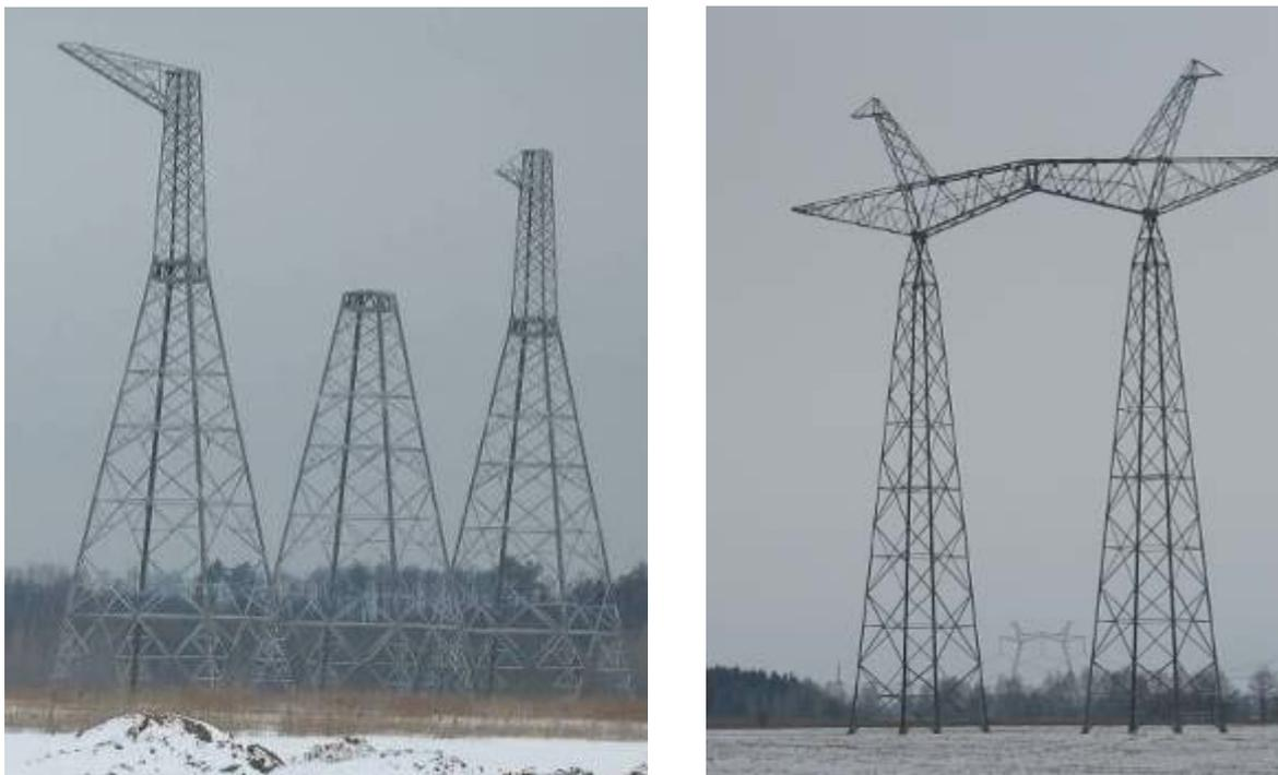
**Figure 1.4** Photographs of angle towers and a support tower
