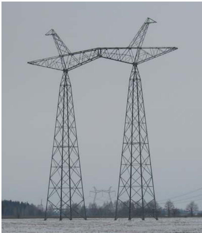
**Figure 6.2** Typical 750 kV suspension tower PC750-3
