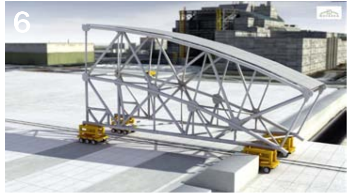
Prefabricated NSC elements transported to site
