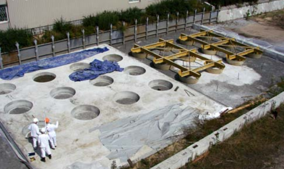
Laying the foundations for the New Safe Confinement
