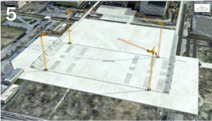
Lifting cranes and sliding pad elements installed
