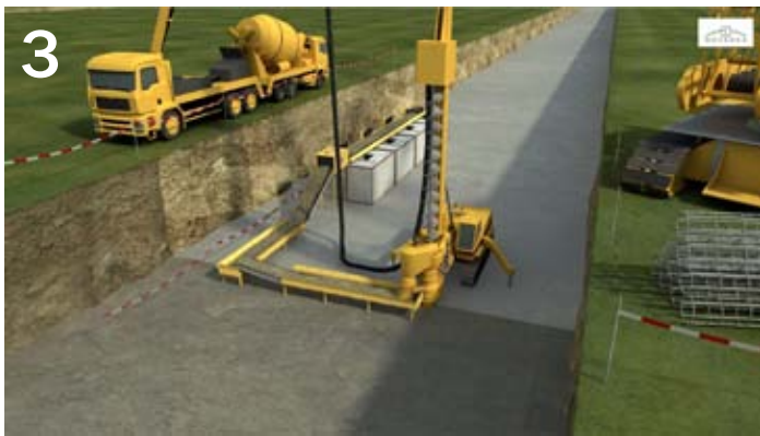
Piling for NSC foundations (current stage)
