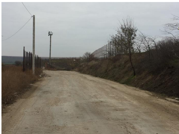
Photo 5: Litter netting that has been installed
