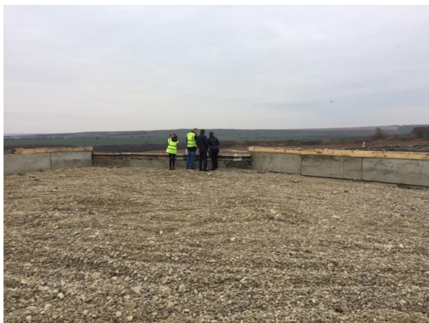
Photo 3: New tipping platform under construction
