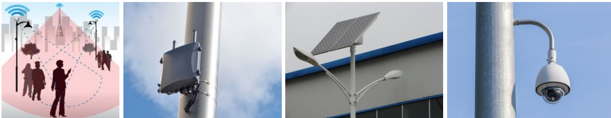
Figure 9: Examples of alternative usage of street lighting poles: for Wi-Fi hot spot, 4G telecommunication, solar panels and video surveillance cameras
