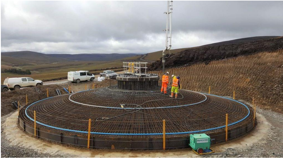
Figure 7: Wind turbine foundation construction
