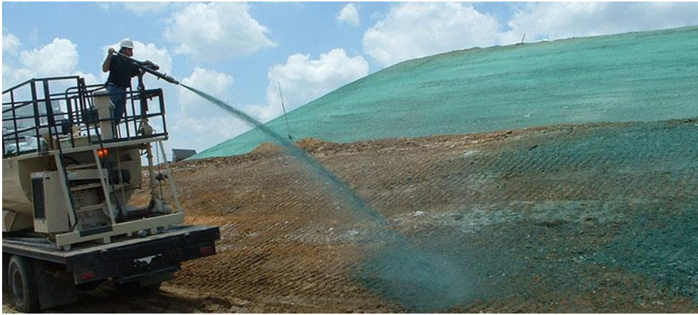
Figure 11: Example of hydroseeding used for reinstatement activities
