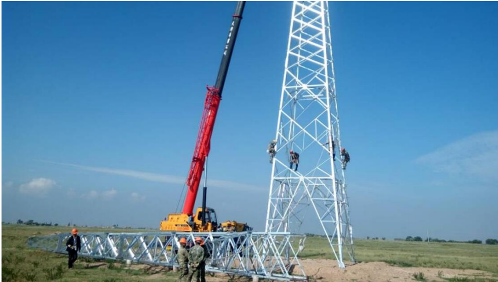
Figure 5: 110 kV pylon assembly
