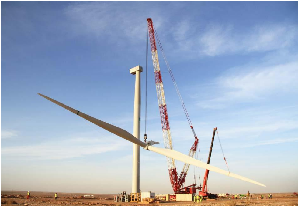
Figure 10: Wind tower assembly
