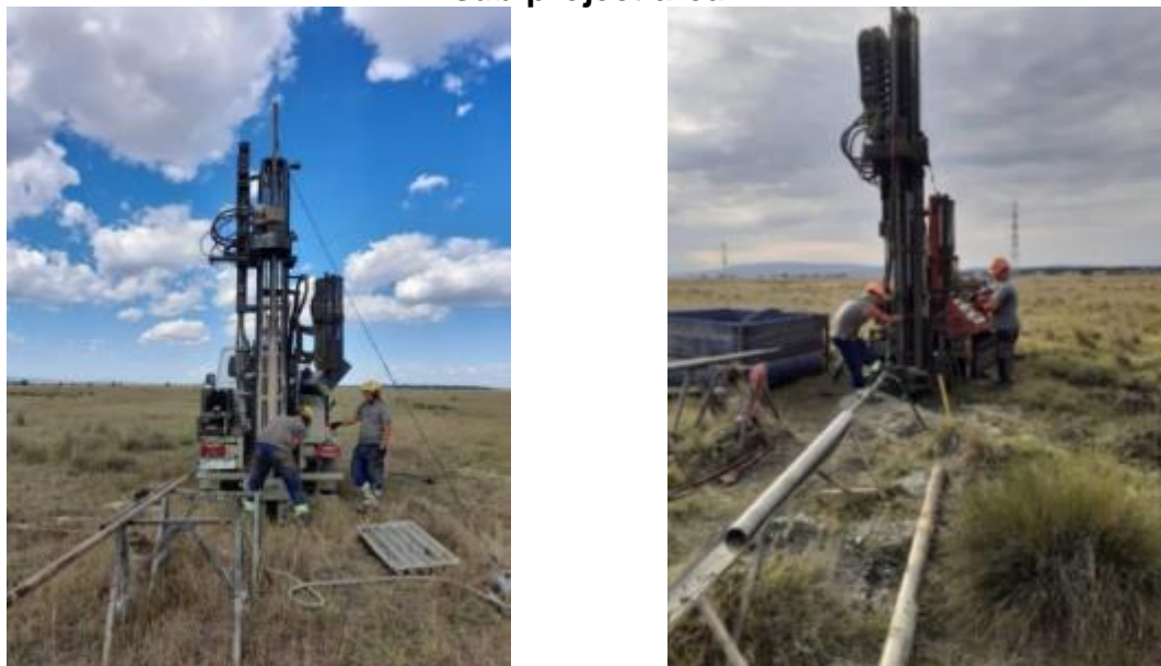
Figure 6-12 Geotechnical drillings at WTG03 and WTG04 locations, Costești sub-project area
