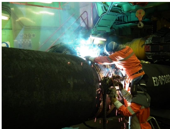
Figure 6-45: Pipe Welding on the S-Lay Barge
