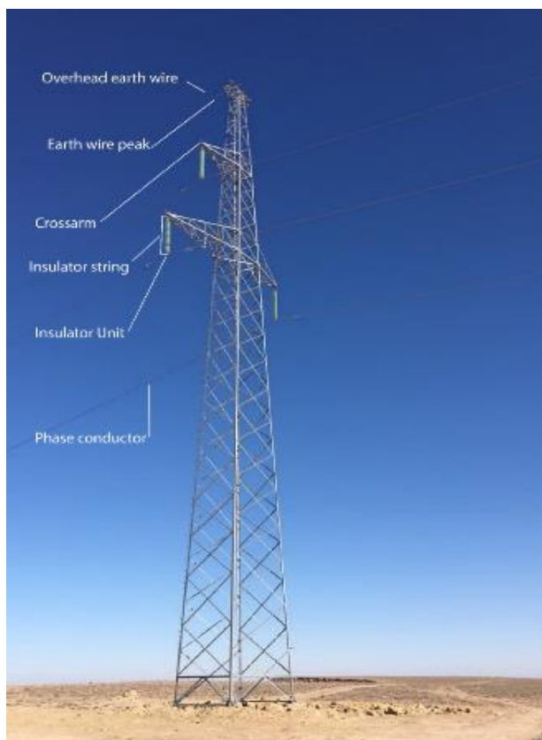
Figure 14: Components of an OHTL (source: Juru)
