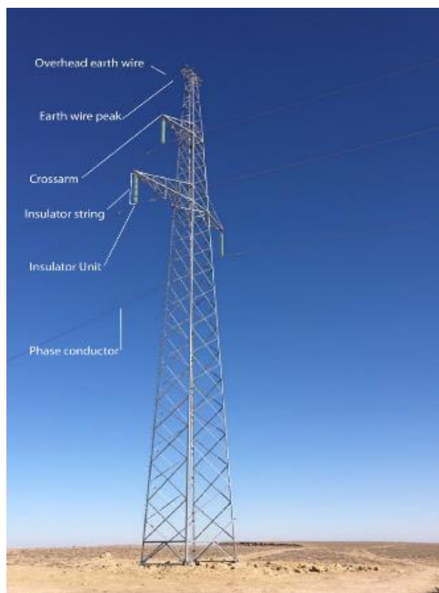
Figure 3: Components of an OHTL (source: Juru)
