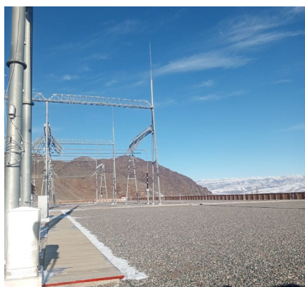
Figure 3: Spare bay for the 500 kV Kemin-Balykchy OHTL in the Kemin substation (source: Kemin Balykchy inception report, December 2024)
