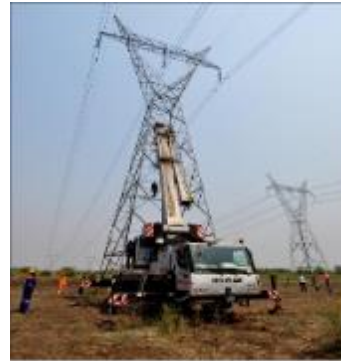
Figure 40: Example of tower assembly process (source: http://cscon.co.za/ and EDM)
