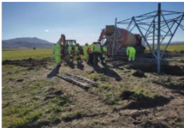
Figure 37: Example of tower foundation construction (source: NJDA, 2022)
