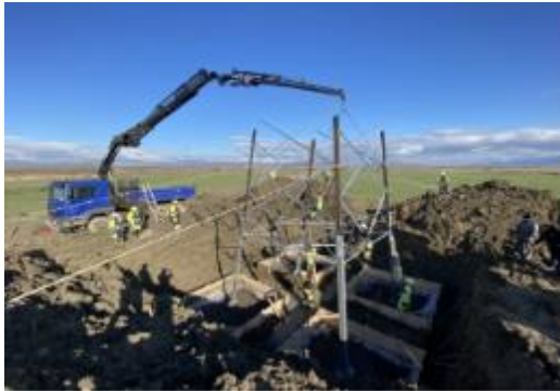
Figure 39: Example of tower assembly process (source: NJDA 2022)
