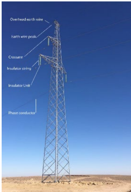
Figure 20: Components of an OHTL (source: Juru)
