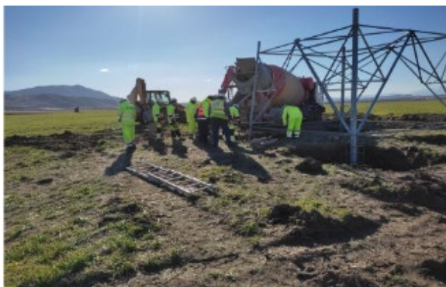
Figure 33: Example of tower assembly process (source: NJDA 2022)
