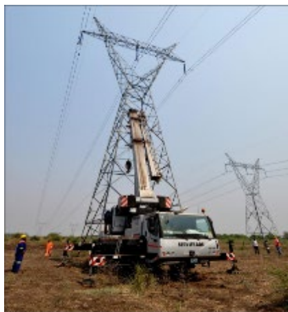
Figure 34: Example of tower assembly process (source: http://cscon.co.za/ and EDM)
