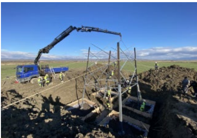
Figure 33: Example of tower assembly process (source: NJDA 2022)
