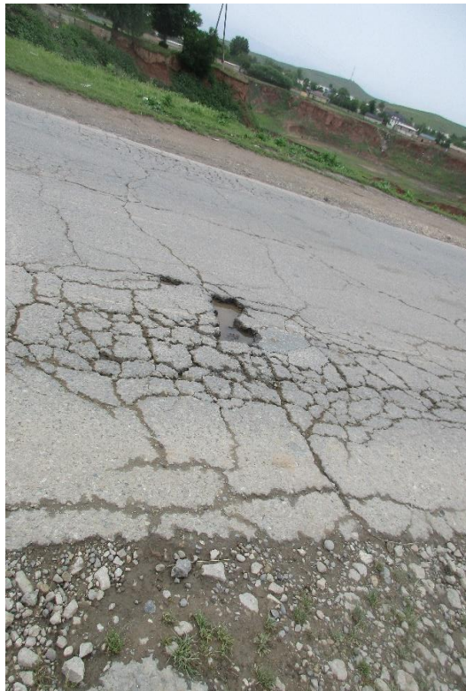
Figure 5 - Severely Damaged Road Pavement (Photo taken 30.04.2024)
