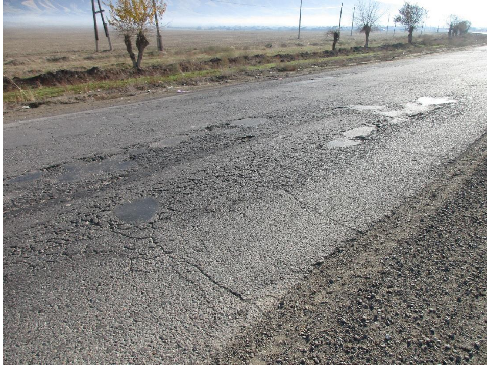
Figure 6 - Severely Damaged Road Pavement (November 2021. Km 17+600)
