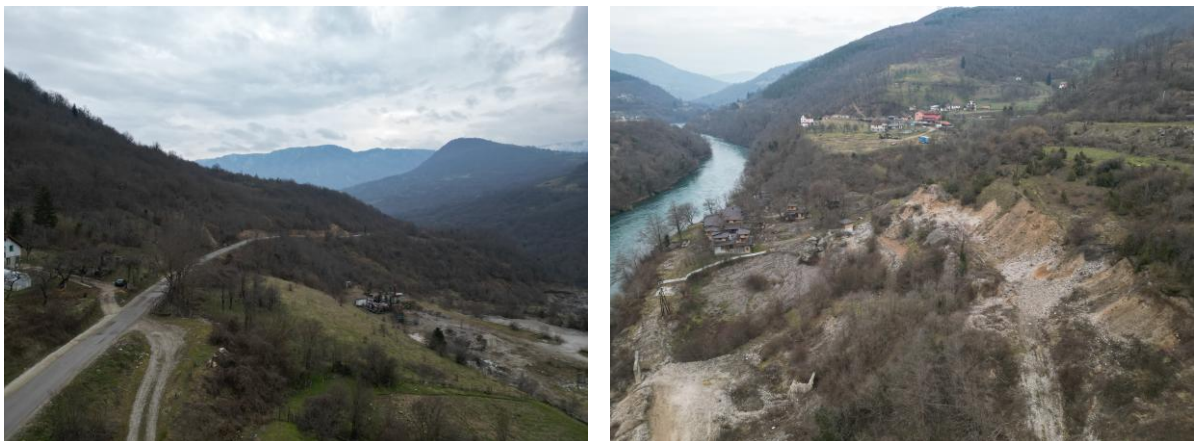
Figure 1: Drone view of parts of the Project area
