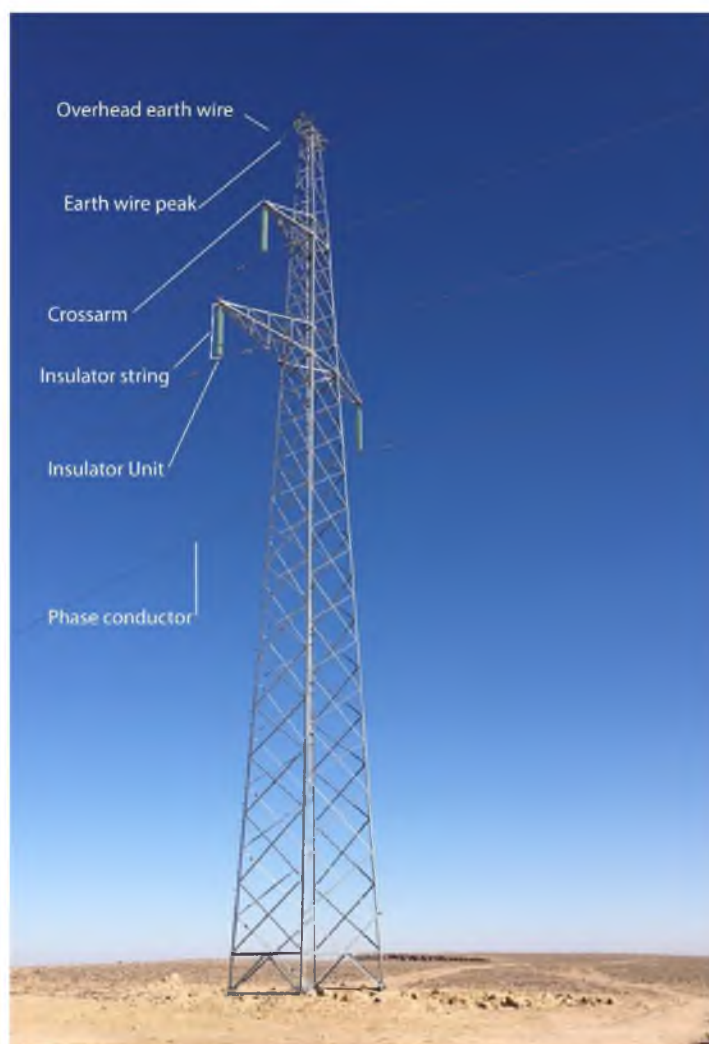
Figure 6: Components of an OHTL (Source: Juru Energy)
