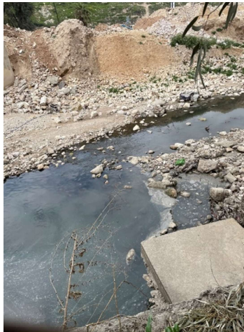
Figure 7: Wastewater Arriving During Storm Events Exceeding the AGTP Peak Design Capacity is Diverted at the Inlet and Discharged to the Adjacent Wadi Without any Treatment in Order to Avoid Flooding the Facilities
