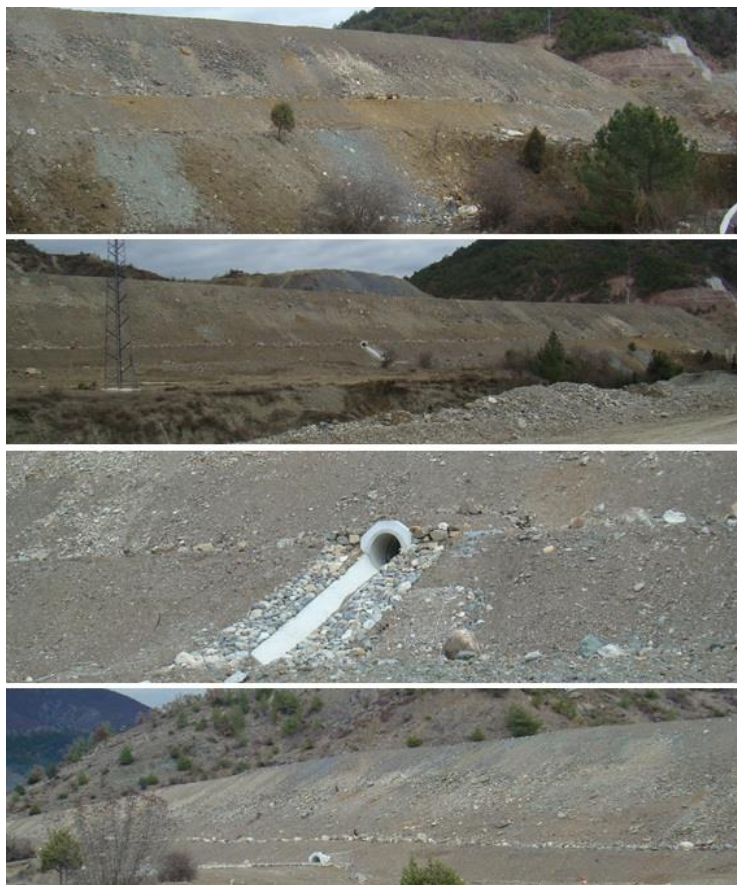
Figure 6-17: Fill Slopes along with Engineering Structures at the GCP Construction Site
