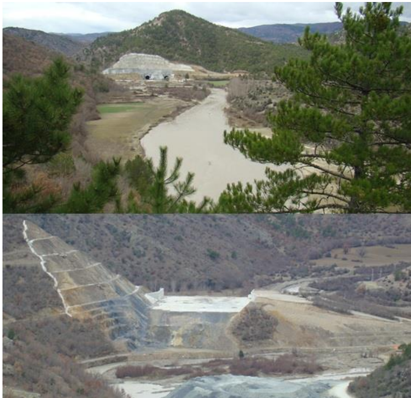
Figure 6-7: Derivation tunnel (top) and Spillway (bottom) Construction at the GCP Mine Construction Site
