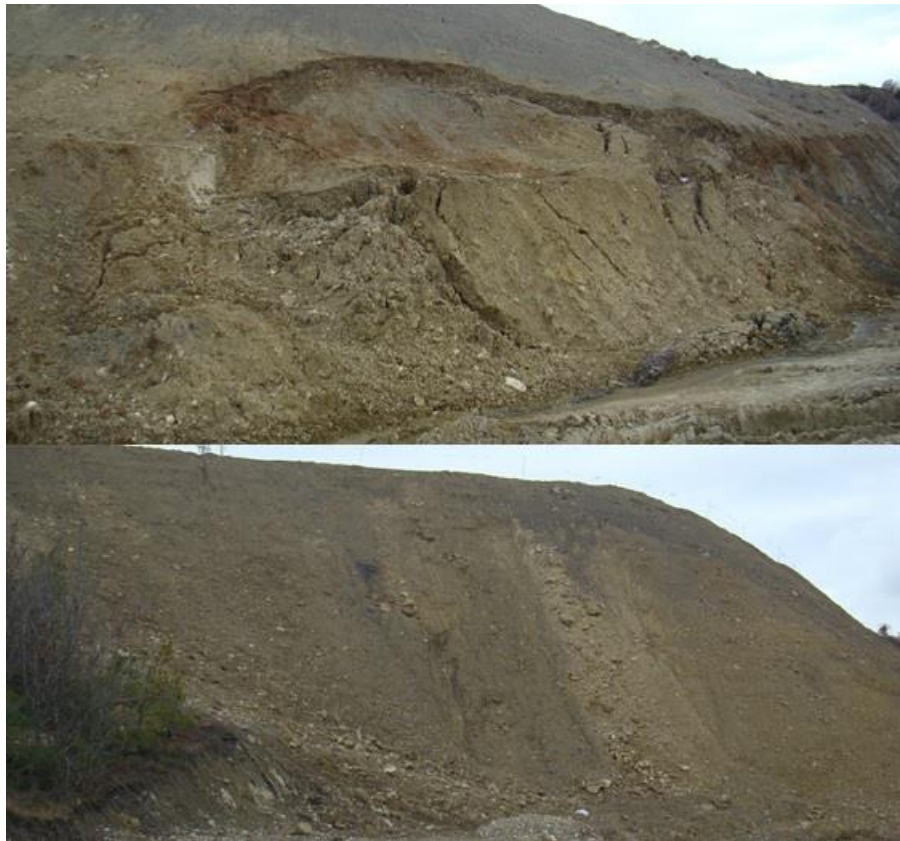
Figure 6-15: Some Mass Movements (falls, slides and flows) on the Cut Slopes at the GCP Construction Site
