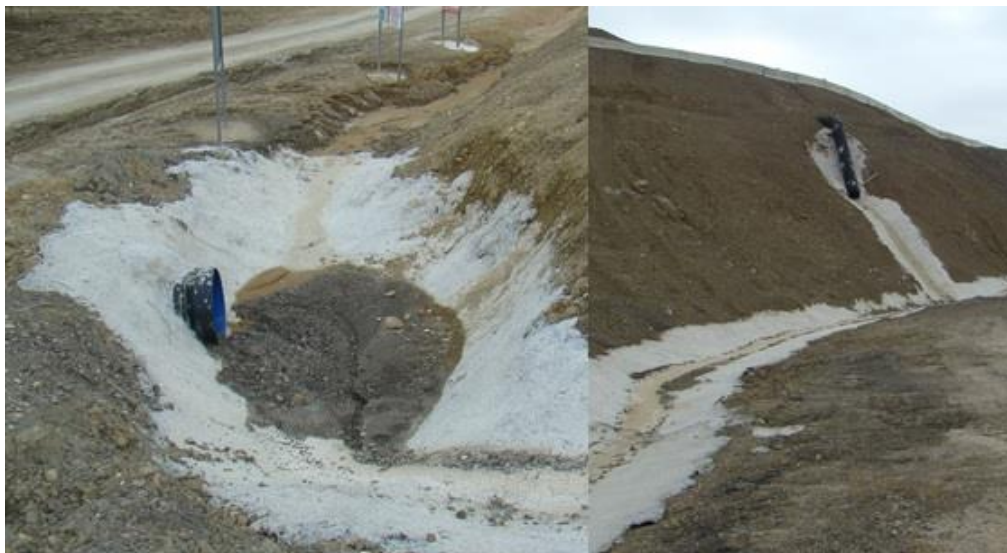
Figure 6-9: Culvert and Toe Ditch (built at a road crossing and along access road cuts)
