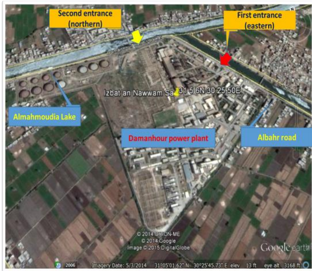
-1:: Entrances to Damanhour Power Station5Figure
