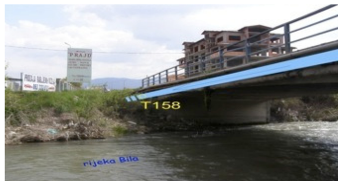
Figure 3. Crossing of the pipeline over the Bila River by suspension
