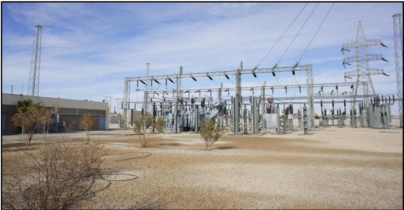
Figure 9: Typical 33/220kV Substation
