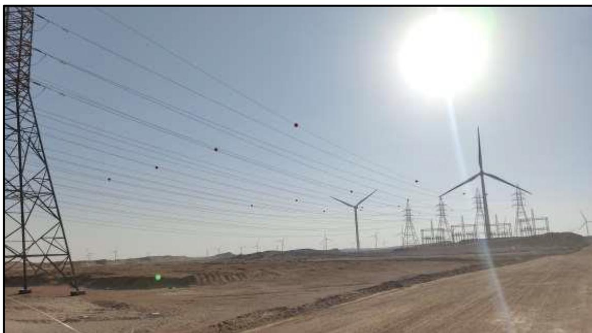
**Figure 107: Bird deterrents on the conductors at RGWE project after Endeco (2023)**
