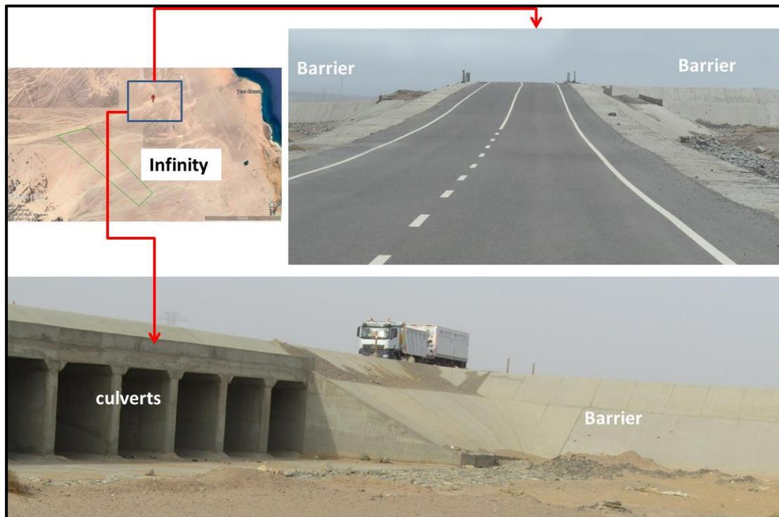
Figure 53: Field photographs show the water barrier at the km 8 and the associated culverts.
