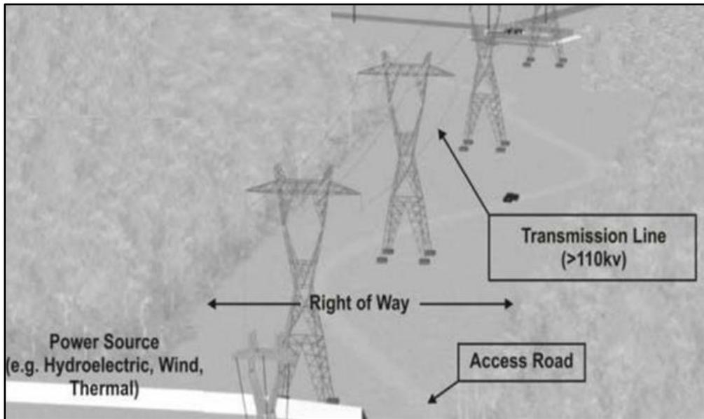
Figure 103: Right of Way and Access Road for OHTL (IFC, 2007)
