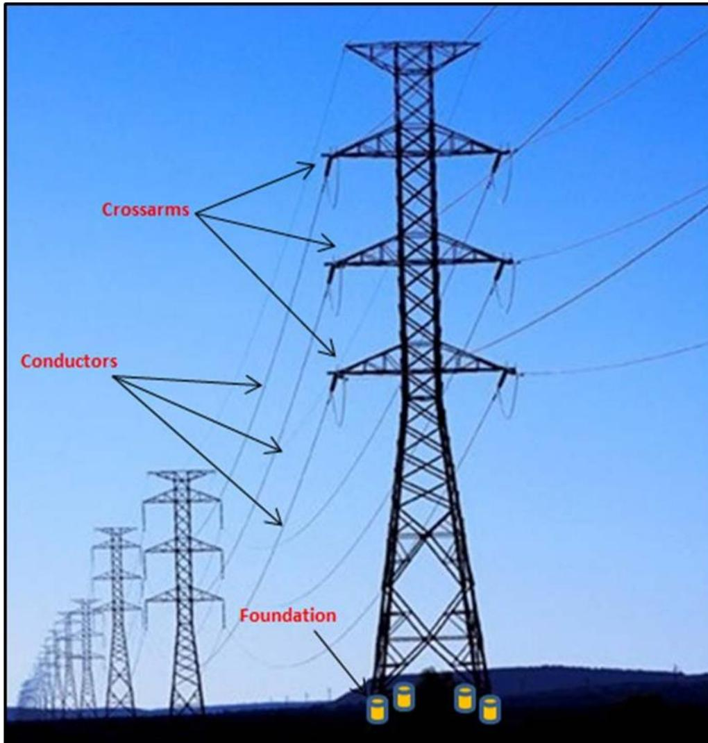
**Figure 102: Typical Structural Components of DCT towers**
