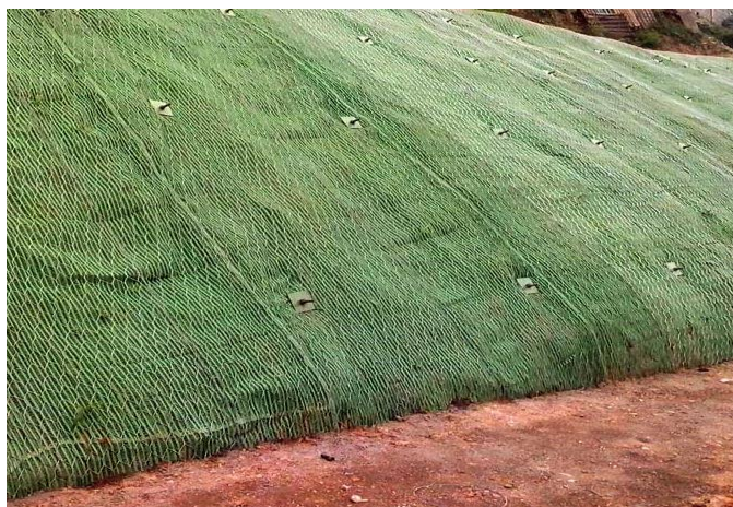
Figure 20 View of principal rock cut stabilization measure by applying regular anchoring, placing of steel wire mesh, and geo-mats
