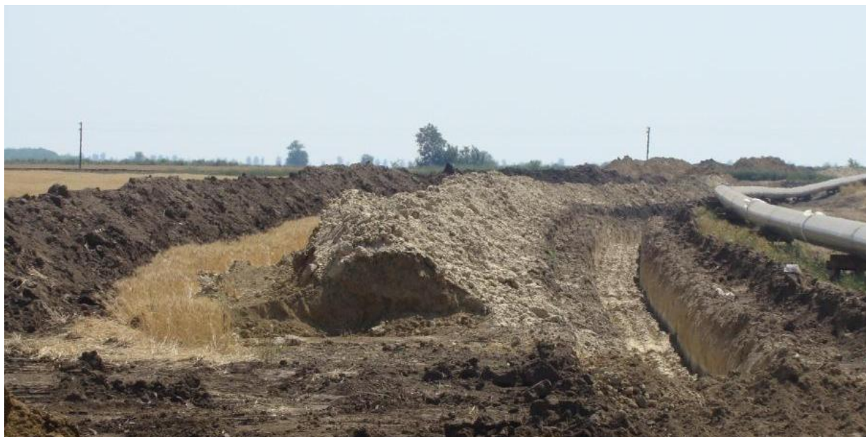
Fig.1.IX. Image of a working strip for gas pipeline laying
