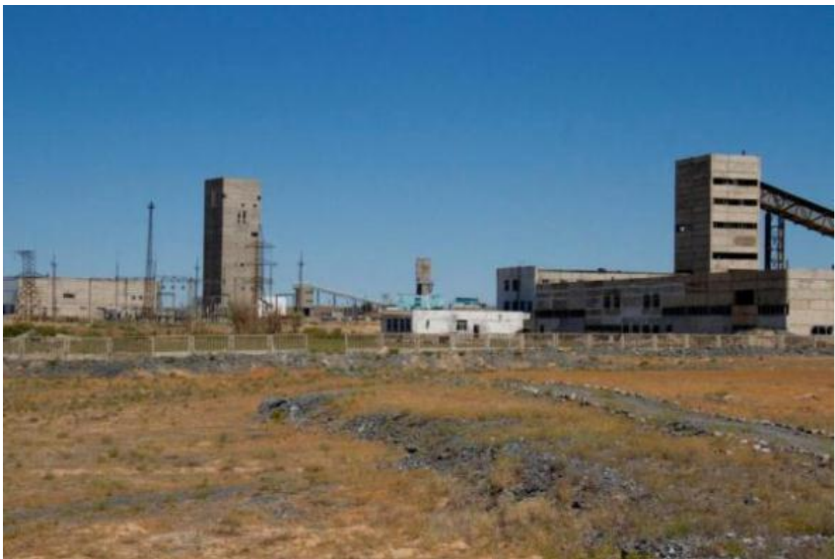
Figure 3: Photograph showing the existing mine infrastructure. The headframe on the forefront (a complex of the Main shaft facility) would be used for hoisting of ore from underground workings using a vertical conveyor
