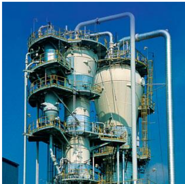
Figure 6. Example of polypropylene unit utilizing Unipol technology (source: https://grace.com/en-us/capabilities/process-licensing )
