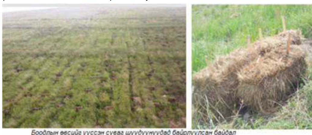
Image 5.20. Hay bales placed at eroded and washed out areas
