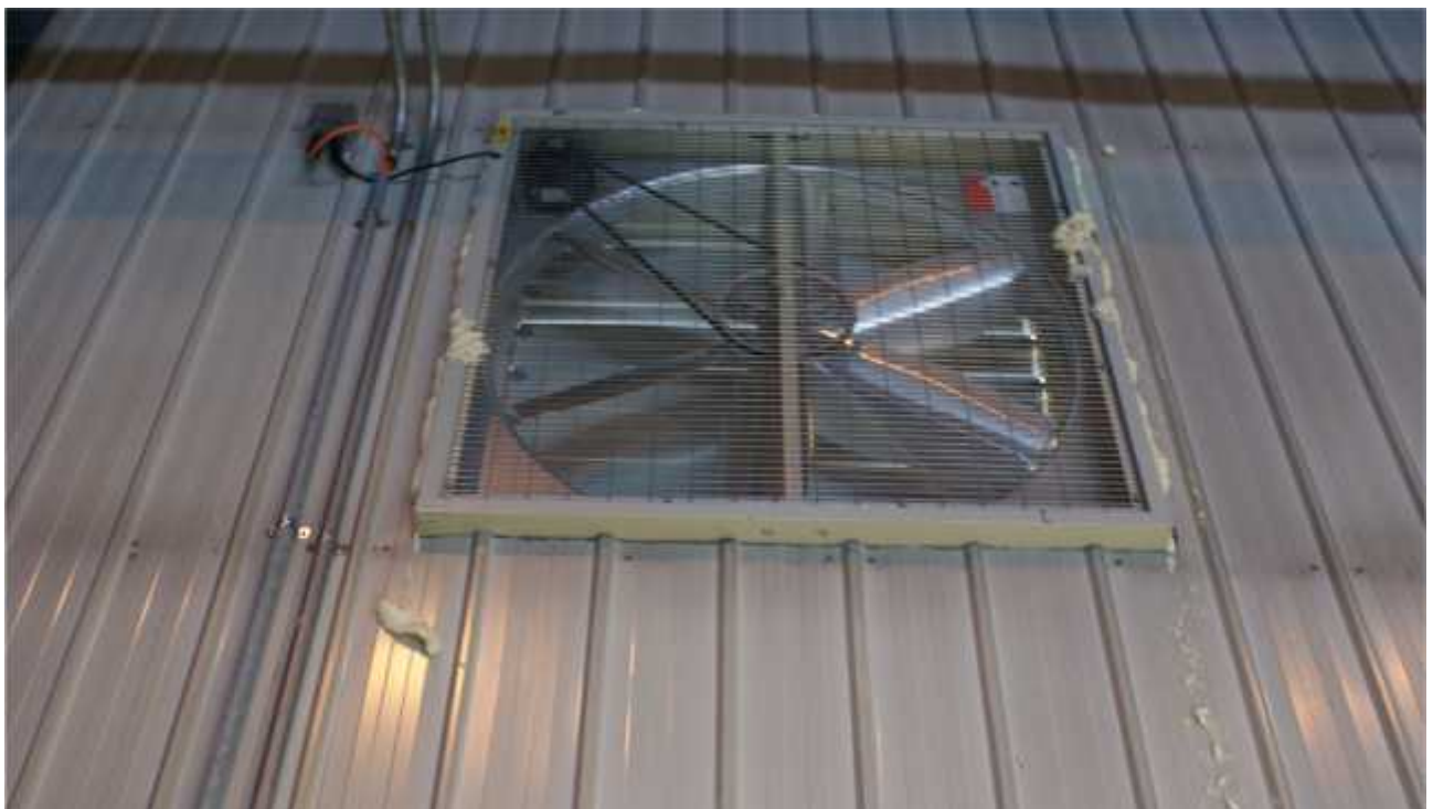
Photo image 4.10 Ventilator to operate at times of excessive cyanide in air
