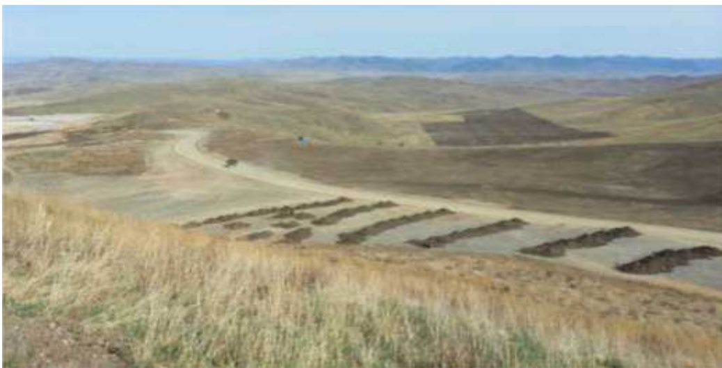
Image 5.5. Topsoil hauled and prepared to spread on area prepared in accordance with standards
