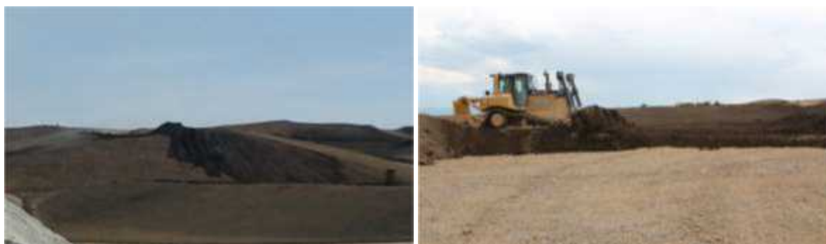
Image 5.6. Spreading and evening the topsoil
