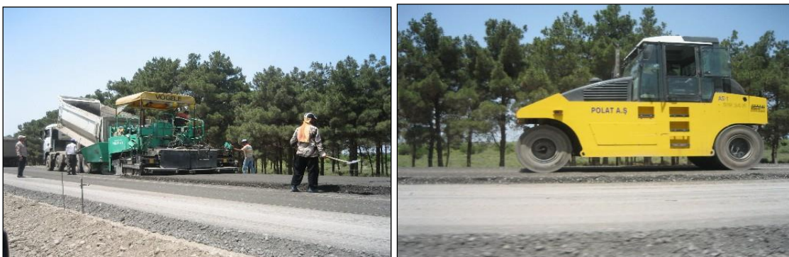
Picture 7: Road Construction along the M-2 Highway. Left shows Road-laying Machine; Right is a Roller
