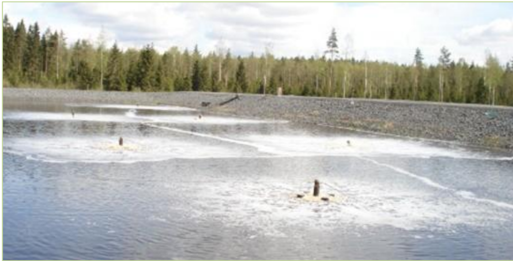
Figure 35 View of an aerated lagoon with surface aerators installed for oxygen supply
