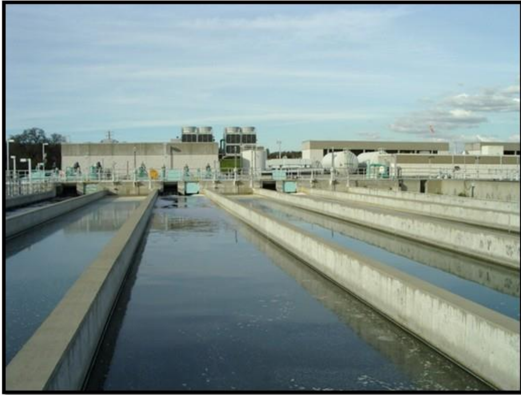
Photo 2 Example of Long Aerated Activated Sludge System
