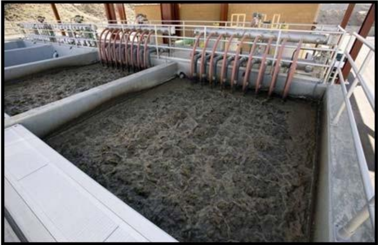
Photo 3 Example of Membrane Bioreactor System
