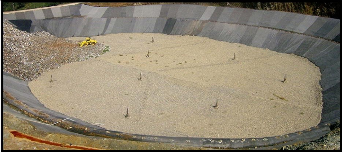
Source: Mezitli Wastewater Treatment Plant Conceptual Design Document, 2013. Photo 4 Example of Storing Treatment Sludge in Regular Storage Areas
