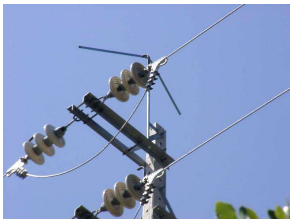
Figure 8-84: Distribution pole with symmetric chevron on top as bird exclusion device.
