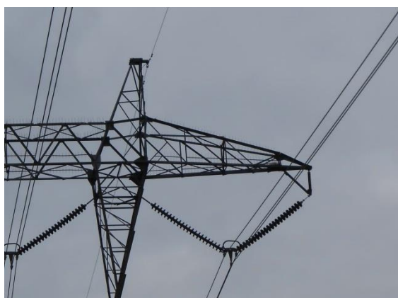
Figure 8-82: existing powerline parallel to the new powerline route with perch discouragers (spikes)
