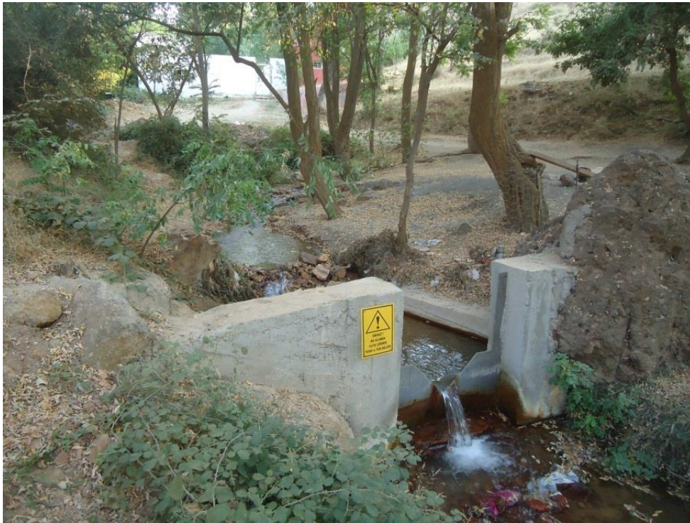
Figure 10-5: Weir Installed on the Öksüt Creek
