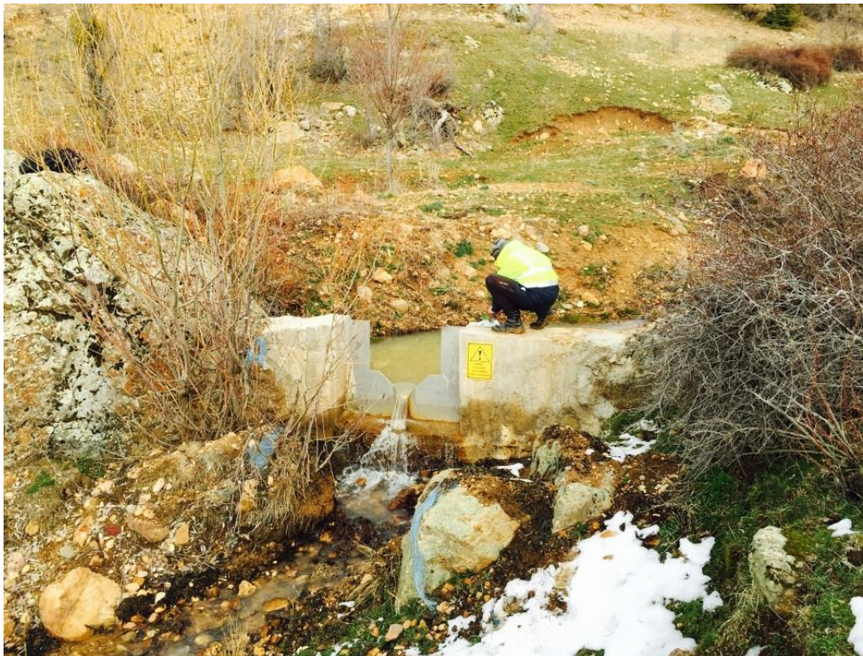
Figure 10-5: Weir Installed on the Öksüt Creek
