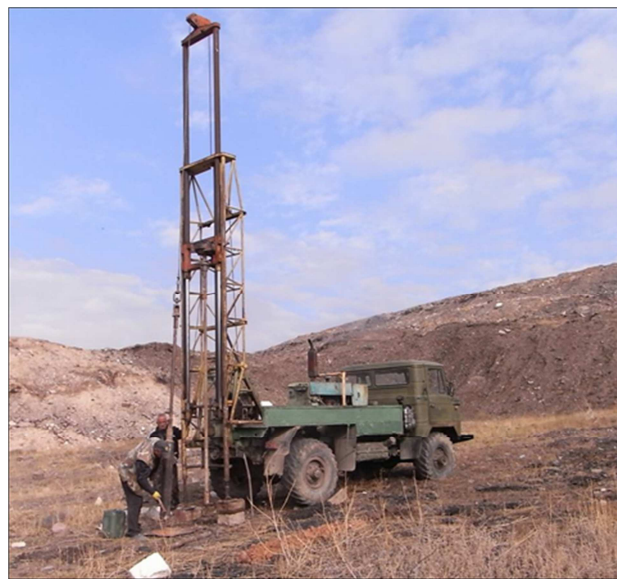
Figure 48: Drilling procedure of boreholes on new landfill area in Oct 2014
