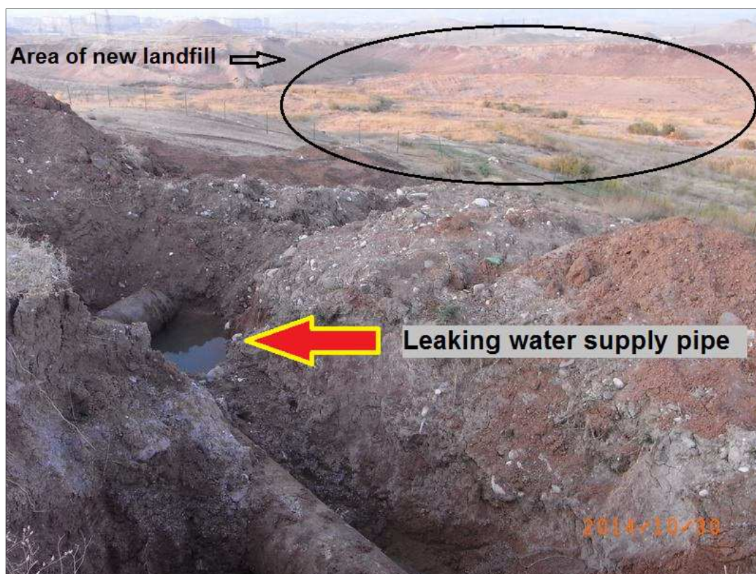
Figure 57: Leaking water supply pipe
