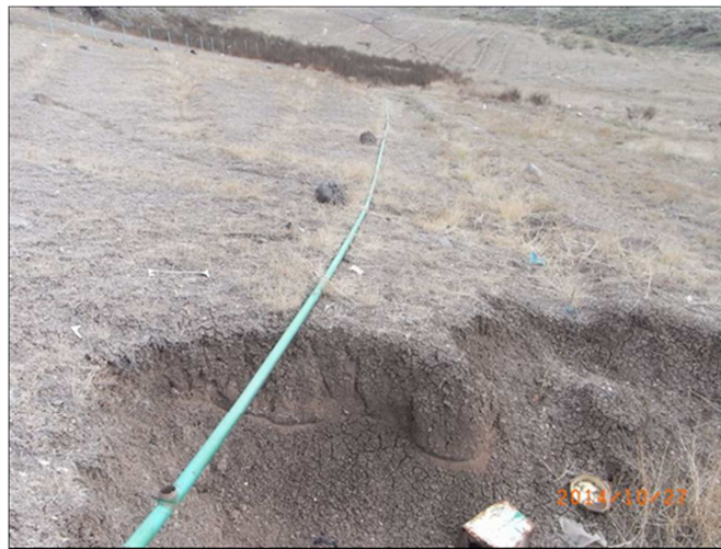
Figure 58: Extensive erosion caused by water from irrigation pipes
