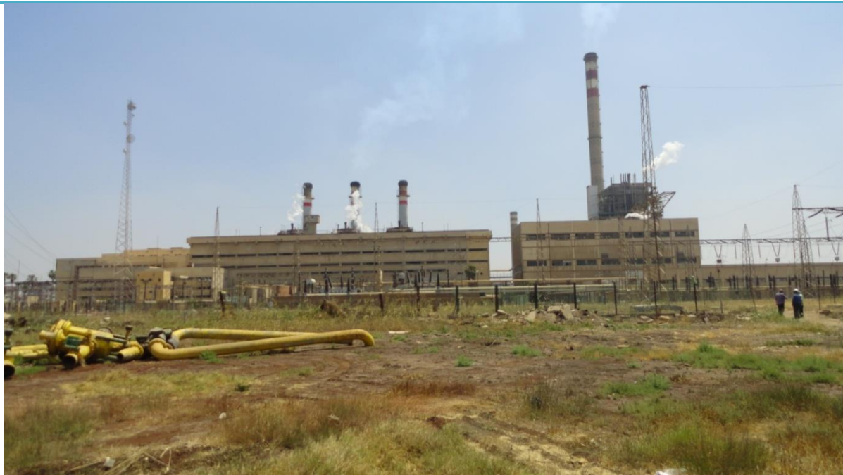
Figure 1-4: View of the main units. The 3x65 MWe units are on the left, the 300 MWe unit is on the right (stack height 138 metres). The 3x65 MWe units are to be decommissioned and demolished simultaneously with the NDPP commissioning.
