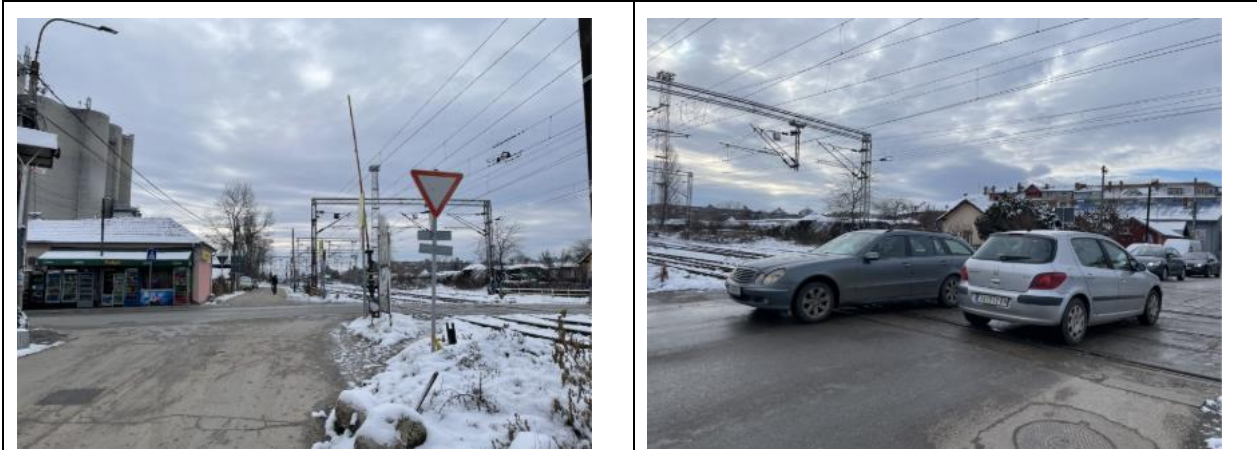
Figure 5: Kapetana Koce Street level crossing (subject to closure under the initial alignment)
