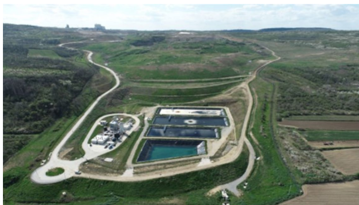
Vinca landfill leachate treatment plant. Source: Beo Čista Energija
