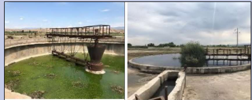
Sedimentation tanks
