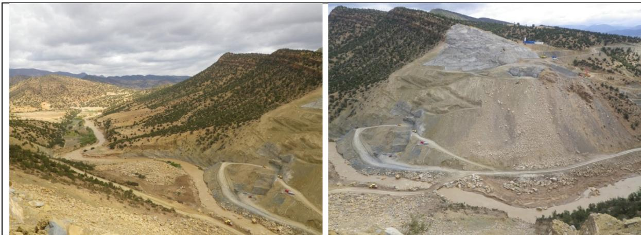
***Picture 4 – Views of the construction site – early 2016: access roads were built, left and right bank abutments were prepared and underground works were ongoing.***
