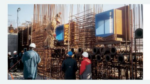
Construction work on the Chernobyl decommissioning facilities is progressing well, with civil works on the Liquid Radioactive Waste Treatment Facility (LRTP) almost complete.
