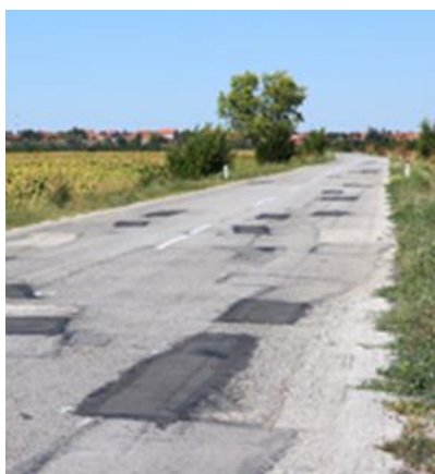
The Serbian Road Rehabilitation and Safety Project is expected to have a systemic impact on inclusion in the country
