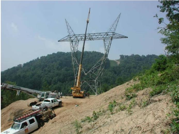
**Fig 3.** Erection of towers
