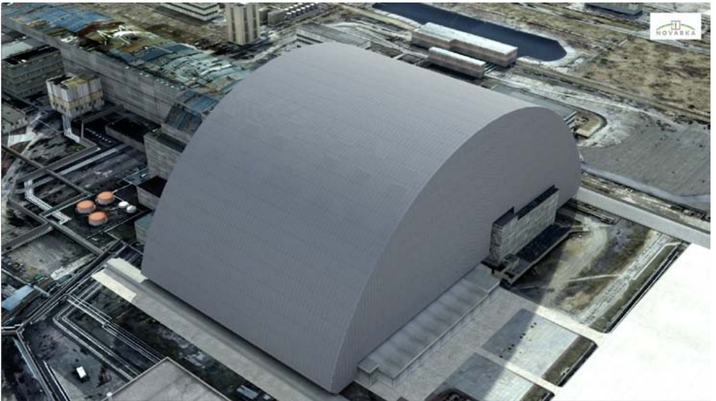
Final structure will cover unit 4 and object shelter for at least 100 years
