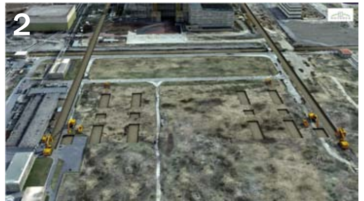
Clearing of NSC assembly area and preparations of lifting tower foundations
