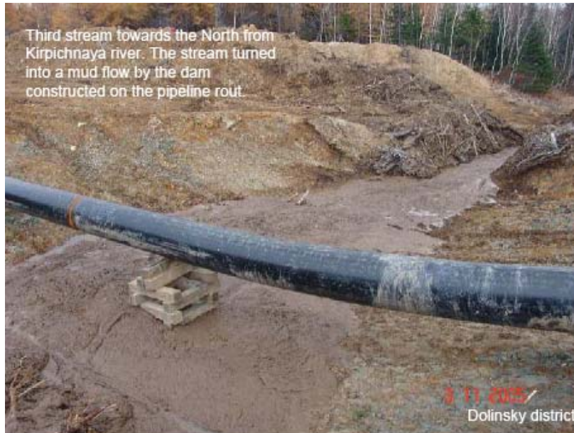
Figure 1 Highly turbid waters with significant plume, even at low flow conditions with small depths (source: Sakhalin Environment Watch photo file, November 2005)
